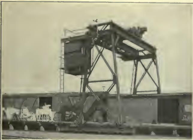
FIG. 317. FREIGHT HOUSES. Gantry Crane at the Wood Street Yard Transfer Station of the Chicago & North Western Railway, 14th Place and Oakley Avenue, Chicago.
